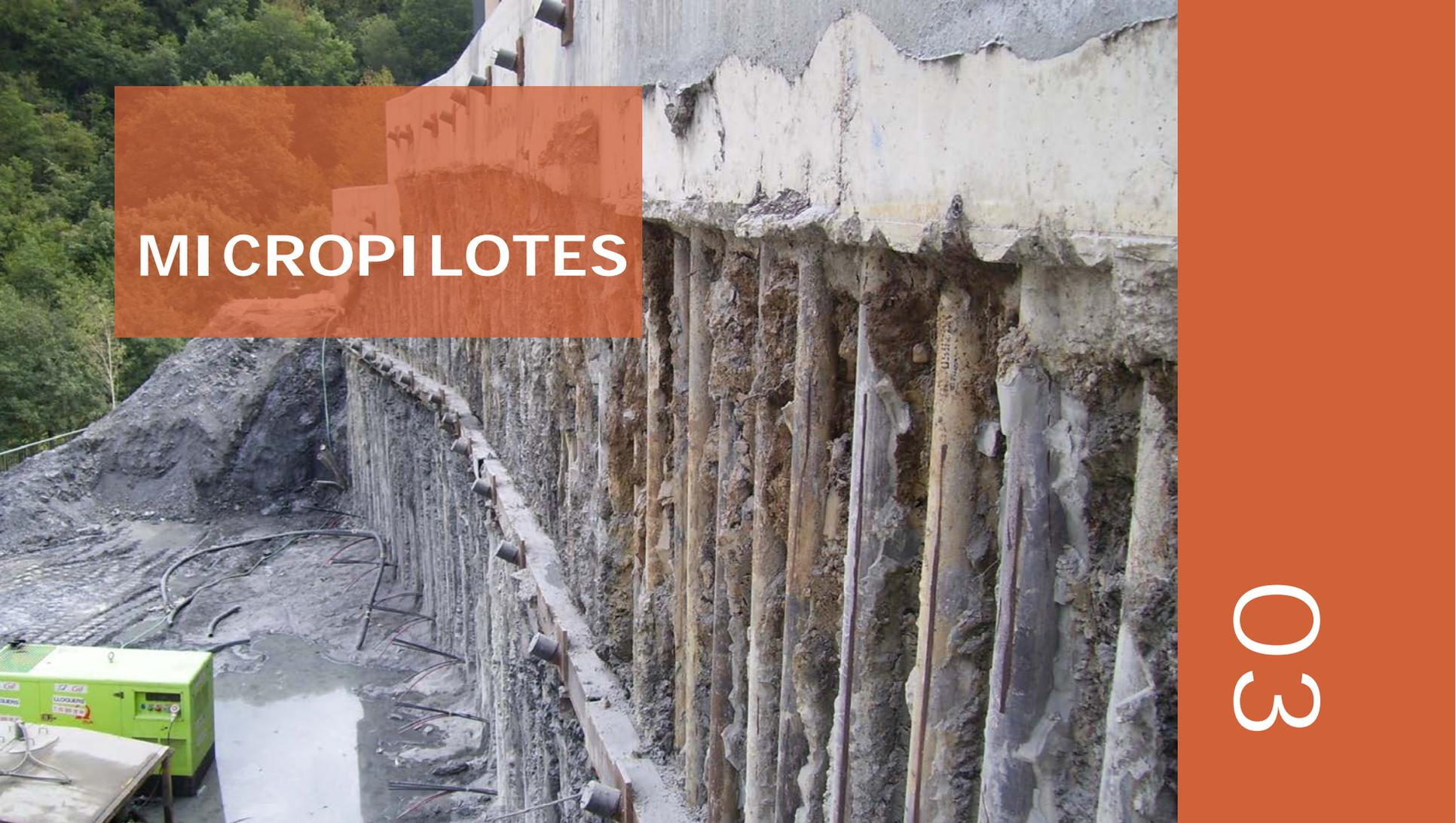
The image shows a construction site for a retaining wall. The wall is made of concrete and has several vertical micropiles installed in the soil. A green generator is visible in the lower left corner. The background shows a steep, rocky slope with some vegetation.
